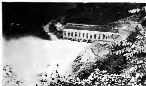
Relief valves of 8,000 h.p. wheels discharging under head of 1500 ft.
